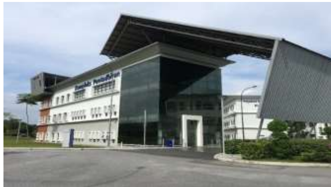
Figure 2: General view of the administration building in the University Technology MARA (UiTM) Tapah
